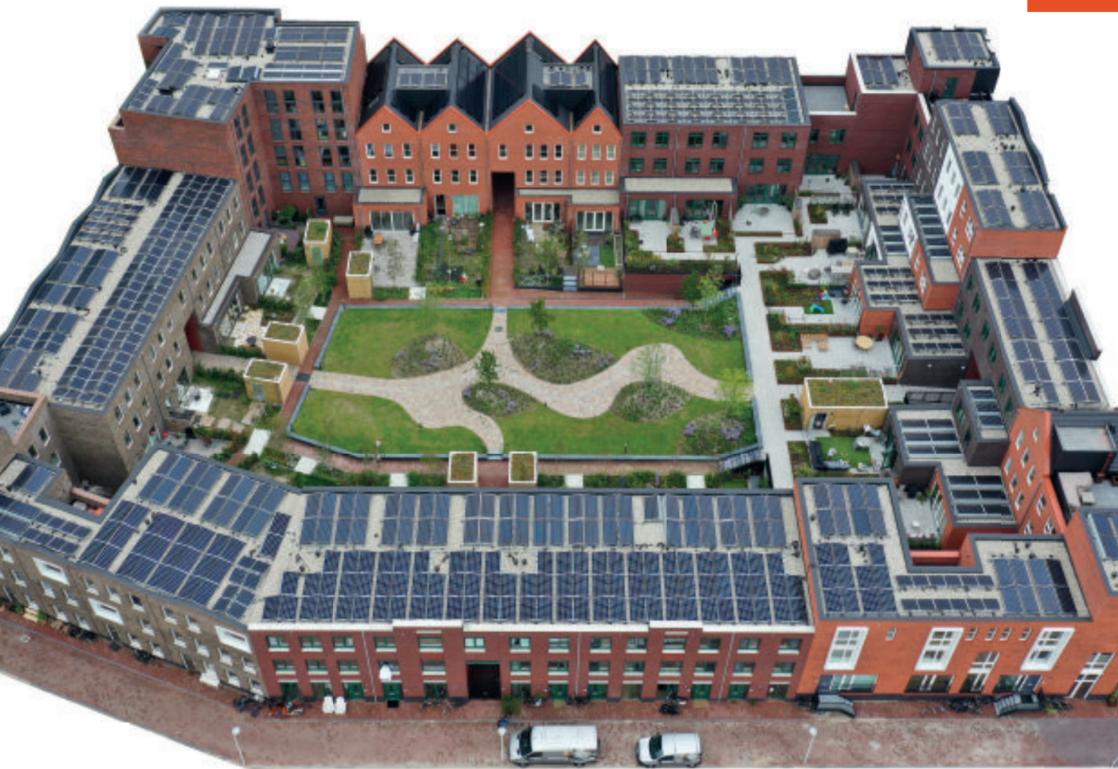
The Ronduit Utrecht Project - 40 energy-generating homes with PVT panels as the energy source
