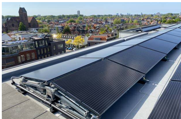
Example of a system on a flat roof of an apartment complex in Delft the Netherlands
