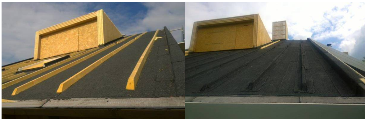
Figure 6.1-a – Wooden beams glued on the bitumen roof.
